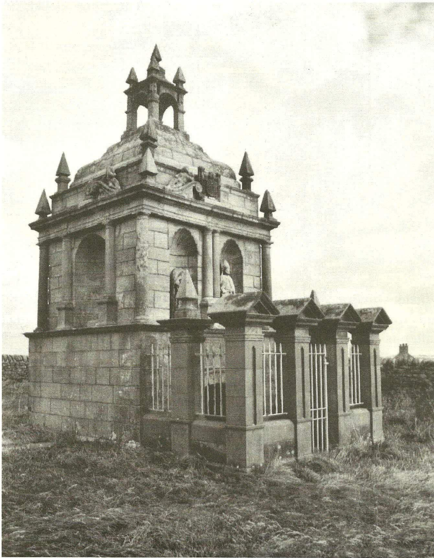
Fig. 5: The Hopper Mausoleum today (railings reinstated by the Churches Conservation Trust)
