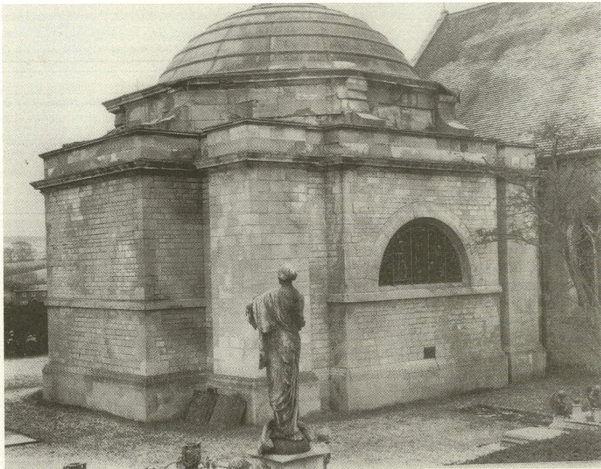
Warter Mausoleum in January 1966, prior to demolition. Photograph RCHM/NMR. Crown Copyright
